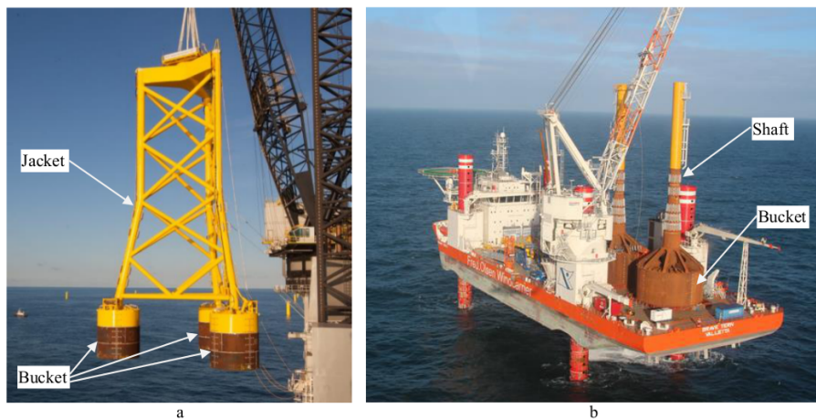
Fig. 1.1: Offshore wind foundations, Kristiansen et al. [2017]. (a) Suction bucket jacket. Photo: Courtesy of DONG Energy. (b) Two mono buckets on a jack up vessel for installation. Photo: Courtesy of Universal Foundation.
