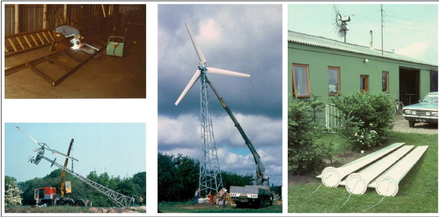
Figure 10: Wind turbine construction in 1978.
