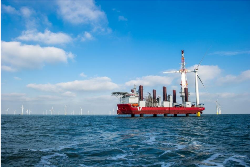
Figure 29: Installation at London Array (2012).
