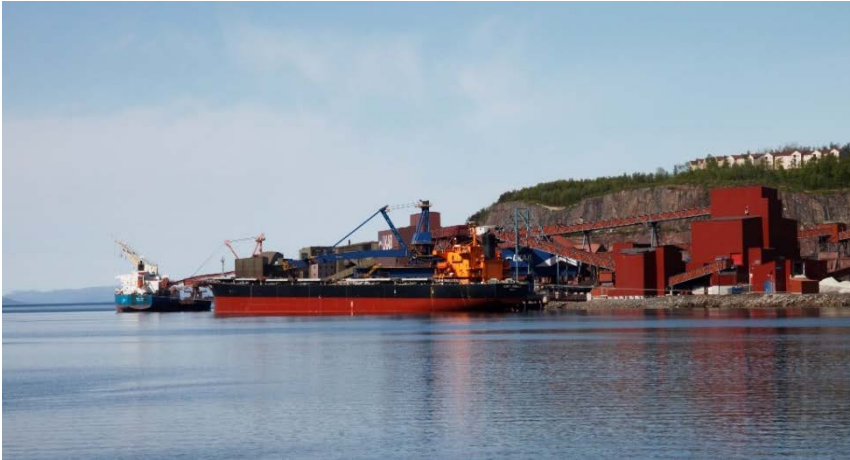
Figure 7. Narvik harbour with both ship loaders in operation (photo: Johanna Fogman)
