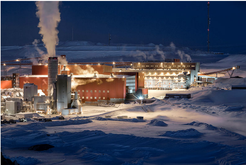
Figure 1. LKAB's newest and largest pelletizing plant in Kiruna (photo: Fredric Alm)
