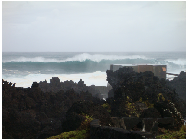
Fig. 2 Waves breaking on the plant the 9/10/2010 at 10:33
