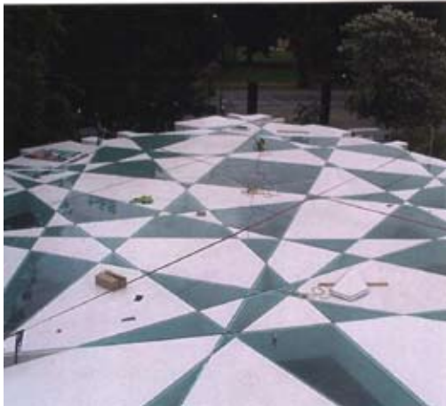
Figure 12-14: Assembly of the Serpentine Pavilion
