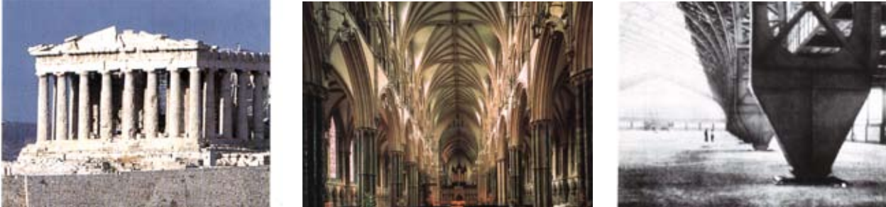
Figure 2-5: The Classic architecture displayed the post and lintel principle. The Gothic architecture used a new structural principle to achieve lightness. The large spans of new building types in the Industrialisation called for new principles.
