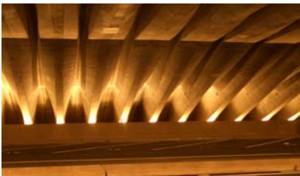
Figure 2: The concourse beams
