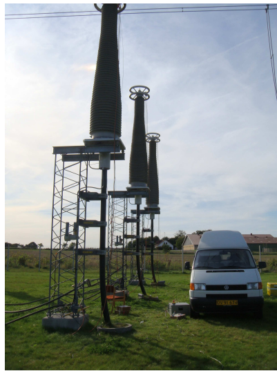
(a) The test setup in Gistrup.
