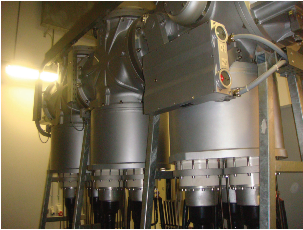
Figure 9.5: A GIS breaker connecting the cable line to its centre placed shunt reactor.
