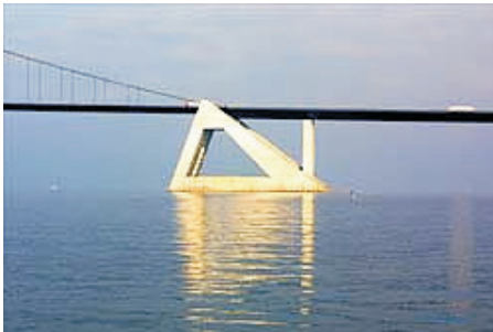
Figure 1.1 An example of a modern large geotechnical structure. One of the anchor blocks of the Great Belt Bridge. ( www.storebaelt.dk )
