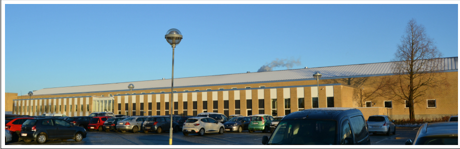
Fig. D.3: Office building used for gathering data. Heating supplied via single mixing loop.
