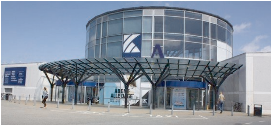
Fig. 1.6: Kolding Storcenter entrance. A Danish shopping center treated in the SEBUT project.
