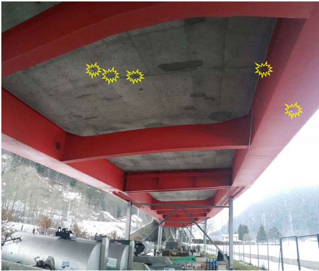
Figure 1. Monitoring system installed on Crêt de l'Anneau viaduct, a view from bottom of viaduct. (Strain gauges locations are highlighted with explosions.)
