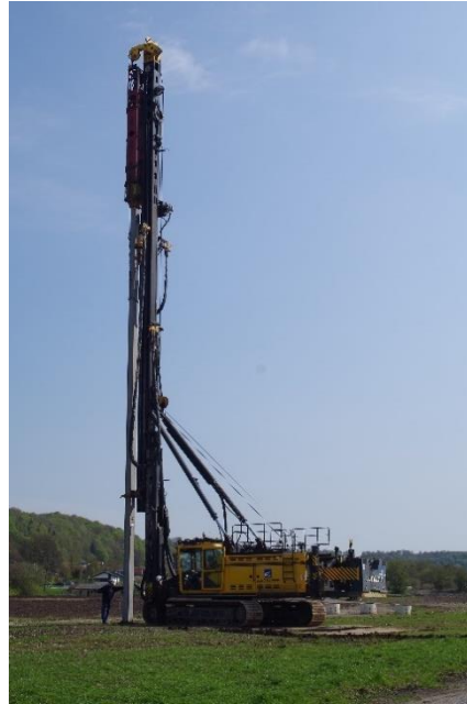
Figure 1-2: a) Demonstration model of the precast energy pile. The concrete has been omitted for illustration. Courtesy of Centrum Pæle A/S. b) 18 m long energy pile driving.
