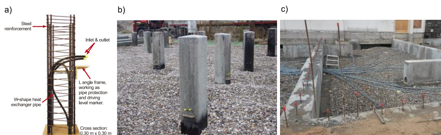
Figure 1: a) Demonstration model of the precast pile heat exchanger with built in geothermal pipes. b) Pile heat exchanger field after driving. c) Pipe work.
