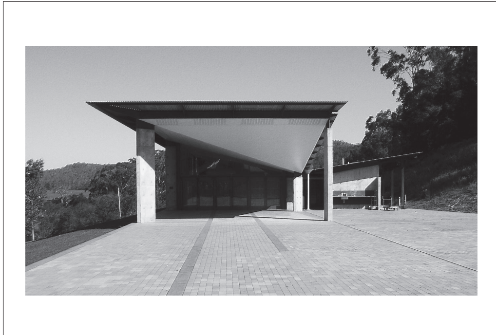
Figure 1.2.1 - Glen Murcutts Bundannon school in Kangaroo Valley Australia
