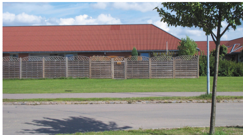
Figure 6.37 Social housing development in the second development zone in the Seden Syd area: Architecture control?
