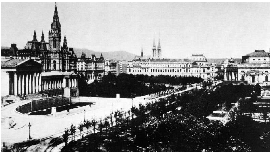
Figure 3.5 Historical photo of the Ringstrasse in Vienna
