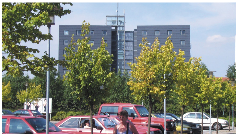
Figure 6.11 Tower block development, seen from the nearby shopping center
