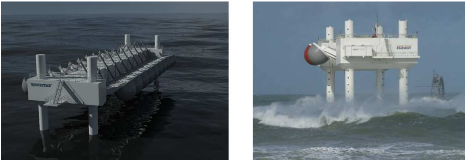
Figure 1.12: Wavestar in storm protection. The right photo is the Wavestar prototype in storm protection, 2009
