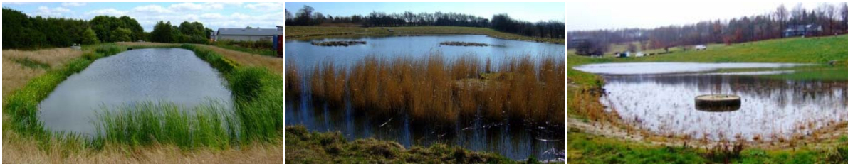
Figure 1: The ponds in Odense, Aarhus and Silkeborg, respectively, approximately one year after construction.
