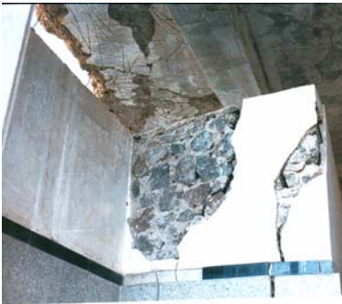
Fig. 432 Inner wall with stone
