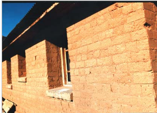
Fig. 422 pre-stressed brick wall
