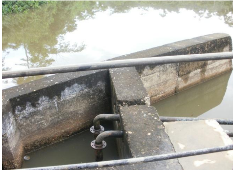
Dammed water from the stream
