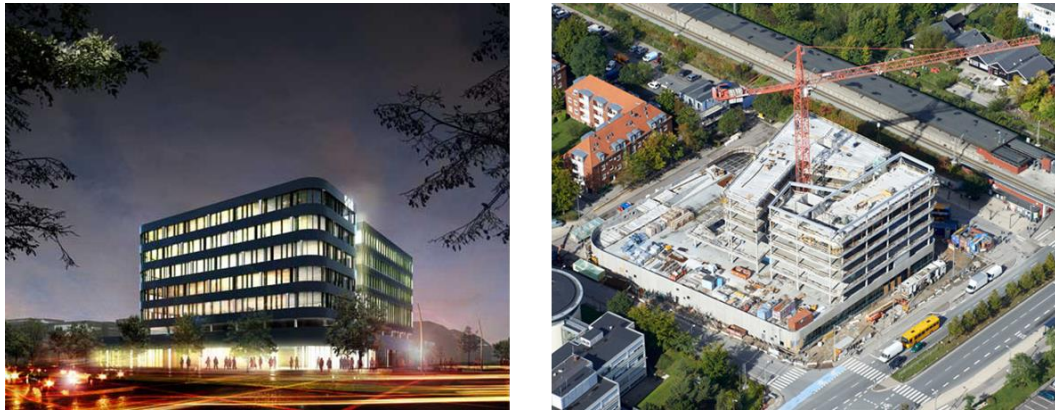
Figure 26: Pictures of case study building.
