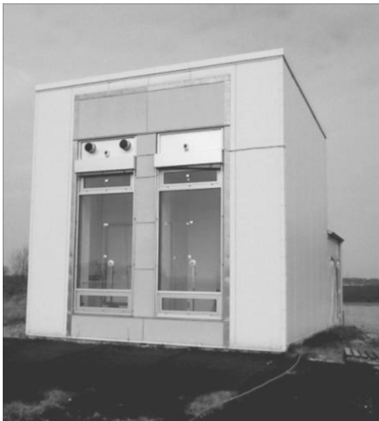
Figure 3: Full-scale façade element test facility.
