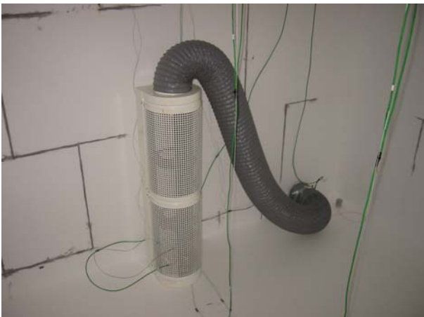
Figure 7. Inlet device for displacement ventilation.
