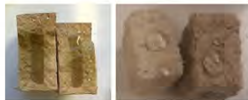
Fig. 13. Penetration depth of agent I on brick and mortar.
