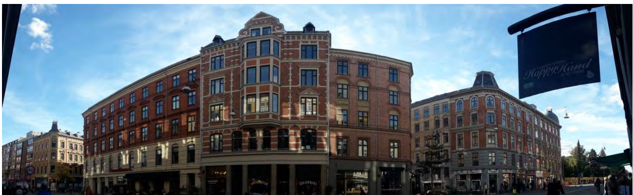
Figure 1: Panorama view of a variety of historic façades of solid masonry facades in Copenhagen, Denmark.
