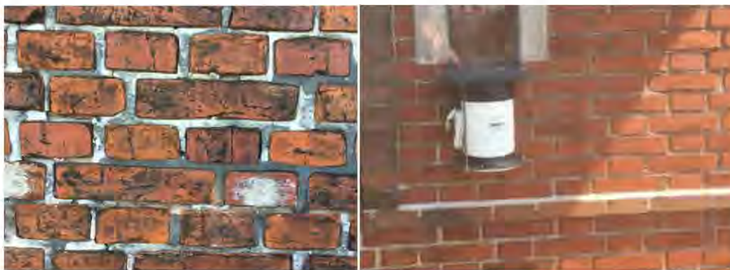
Figure 7: Masonry on façades of test building 1 (left) and test building 2 (right)
