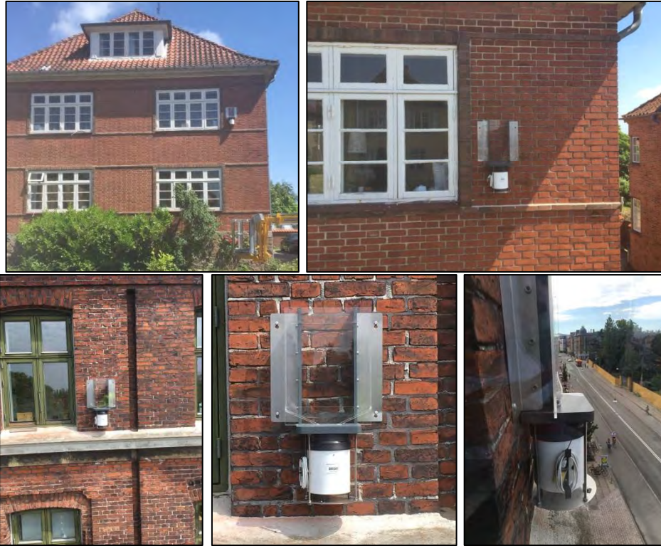
Figure 17: Installation of WDR gauge. Top: Case building 1. Bottom: Case building 2.
