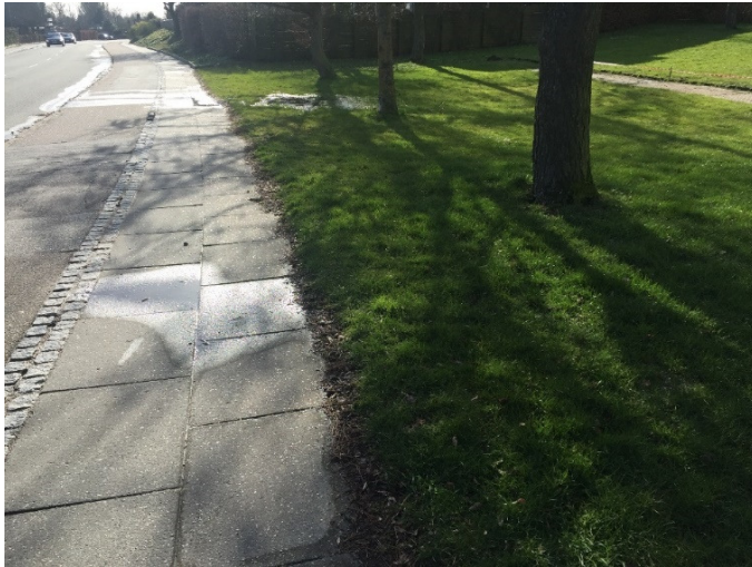
Figure 2.4. Active rainfall-runoff from the experimental location. Discharge occurs although the impervious surfaces are dry.
