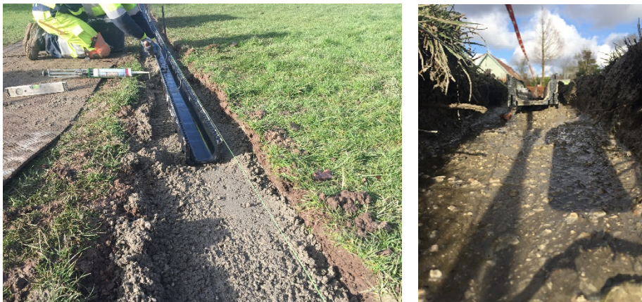
Figure 2.5. Assembling of line drain at the experimental area.
