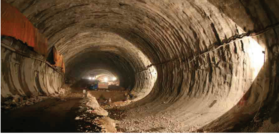
Figure 1.5: Construction of Qingdao Jiaozhou Bay tunnel in Shandong Province, China.
