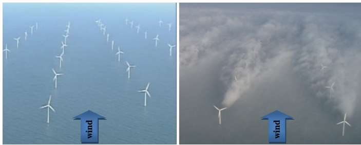
Figure 1.4: The wake of upwind turbines on downwind turbines in HornsRev wind farm.
