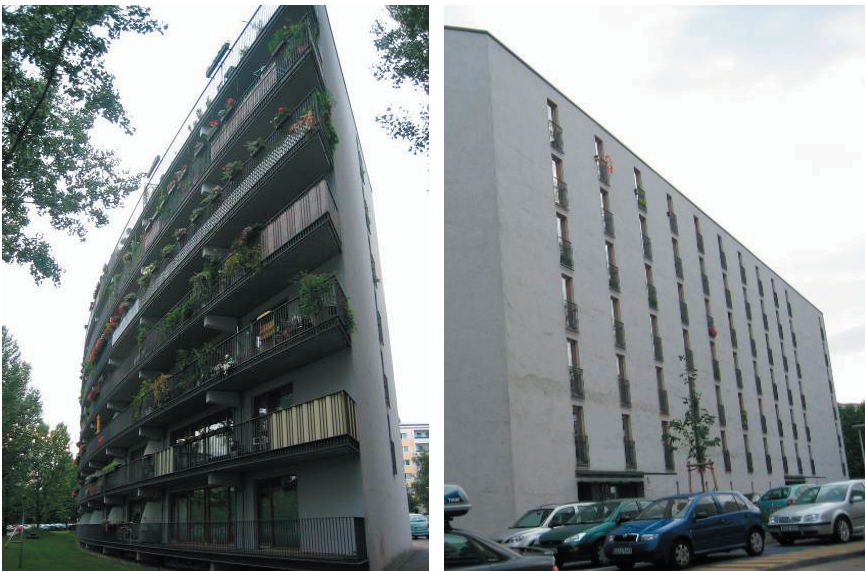
Illustration 118.1: Pictures of the building from 2005 (Left: south facade. Right: North facade).
