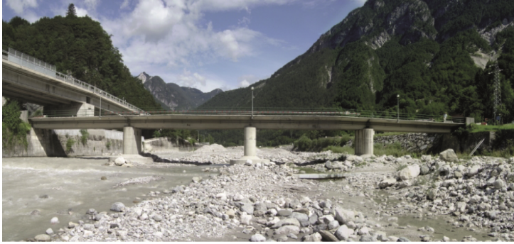
Figure 7.13: Dogna bridge, front view.
