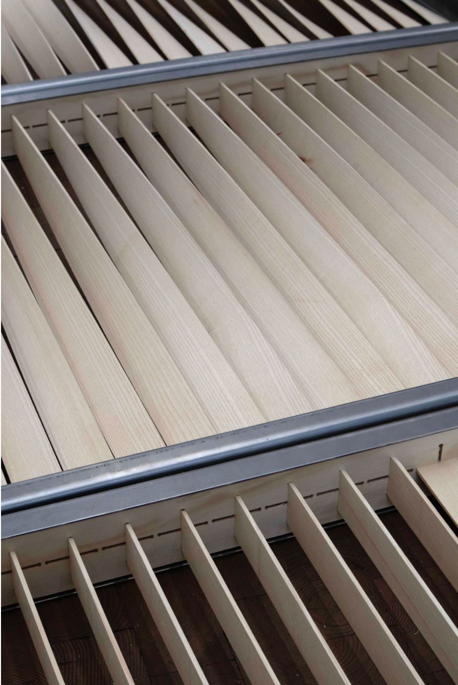
Figure 6.5. Close-up of the wood lamella facade elements. Photo by Avishek Das.
