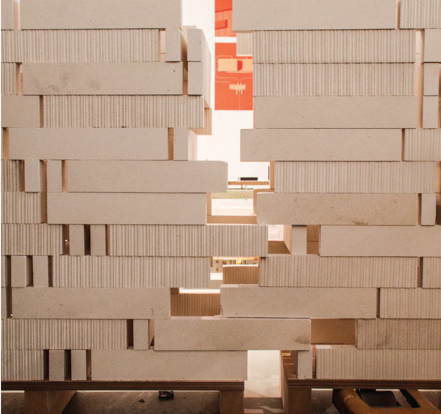
Figure 5.2. The limestone brick wall was produced as four separate section. Here two of the sections are being joined together. Photo by Isak W. Foged.
