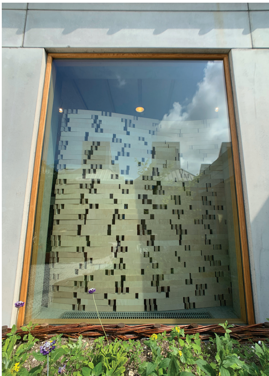
Figure 5.8. Physical demonstrator of the acoustic brick wall. Exhibited in the Utzon Center, Aalborg, Denmark Photo by Mads Brath Jensen.
