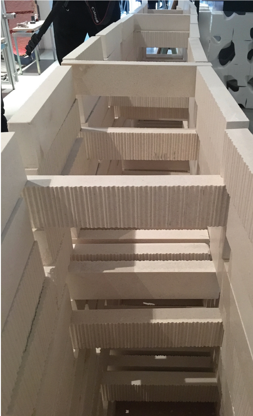
Figure 5.3. The interior composition of the limestone brick wall. Photo by Mads Brath Jensen
