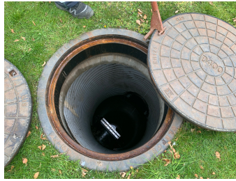
(b) Manhole (Ishøj, Denmark).
