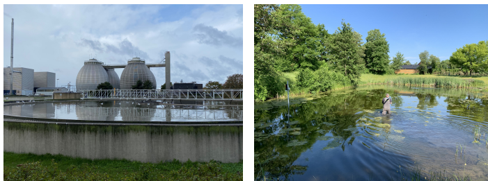
(a) Waste water treatment plant (Biofos, Denmark). (b) Retention pond (Ishøj, Denmark).
