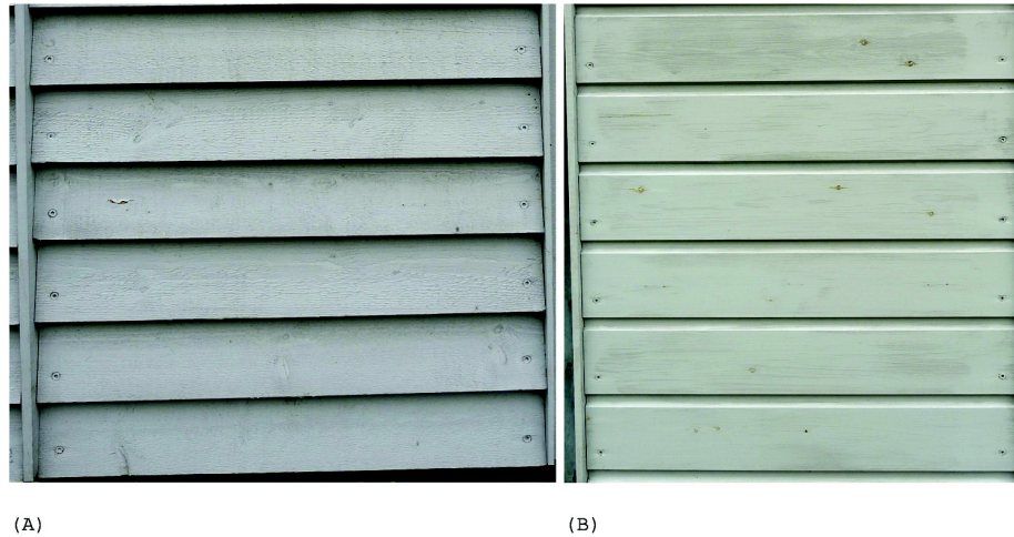
Figure 5 Elements with (A) open cladding (horizontally lapped boarding) and (B) tight cladding (horizontal weatherboard).
