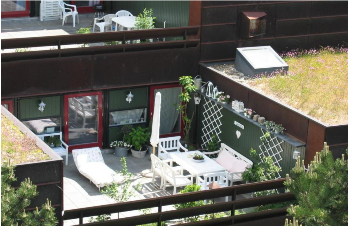
Figure 15: A cozy roof terrace without leaks
