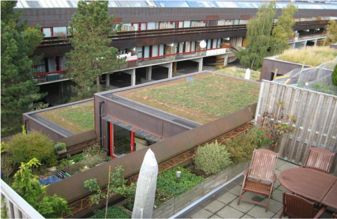
Figure 14: Small vegetative roof systems are visible from the terraces in the apartments above.
