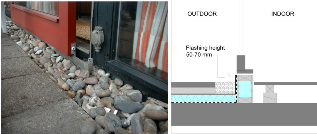
Figure 6: Example of flashings between terrace and apartment
