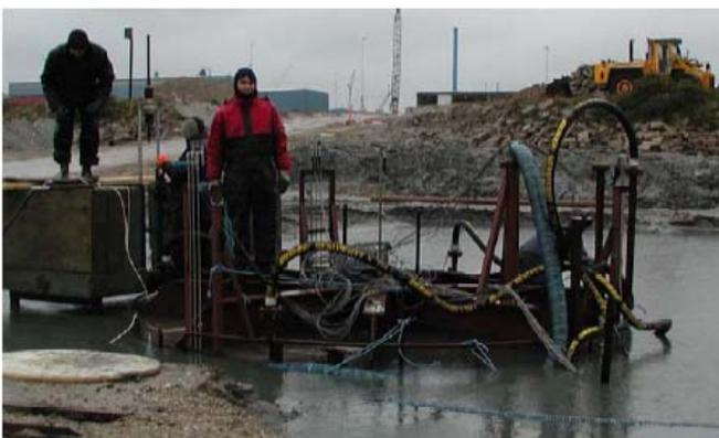
Figure 12. The 4x4m bucket successfully installed.
