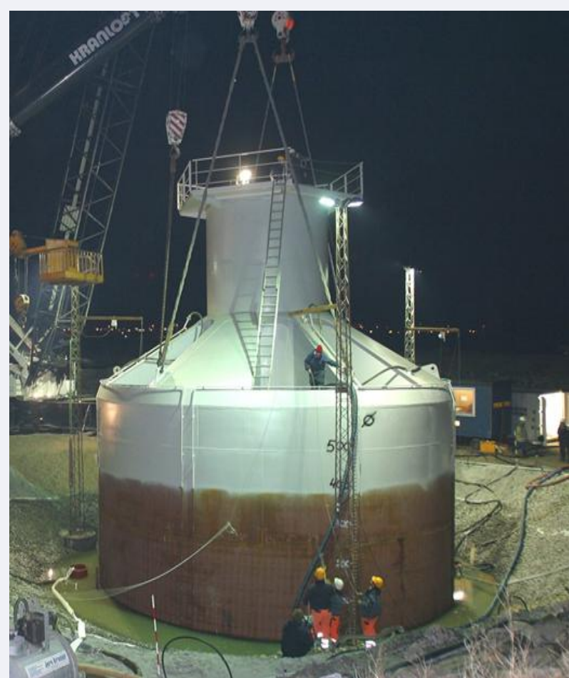
Figure 1: 12 m diameter, 6 m skirt bucket foundation installed in Frederikshavn (DK)
