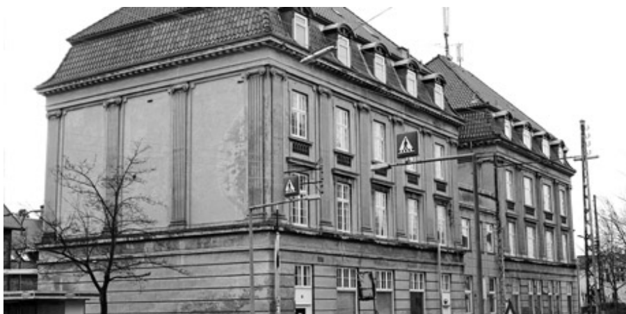
Figure 2. An example of a residential property
