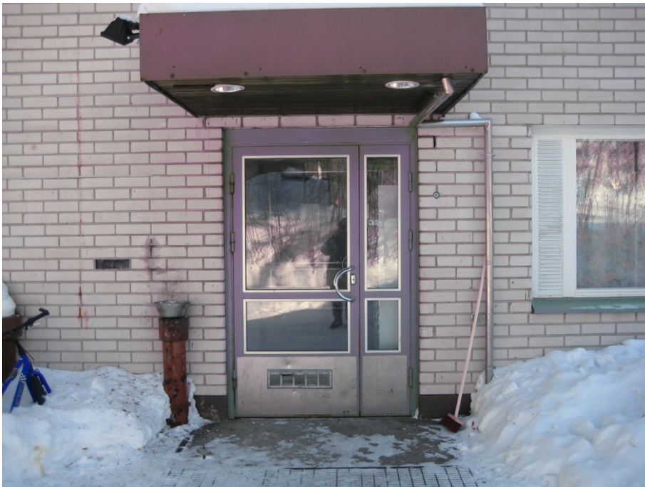
Figure 123. Entrance. Photo: (Jyri Nieminen).
