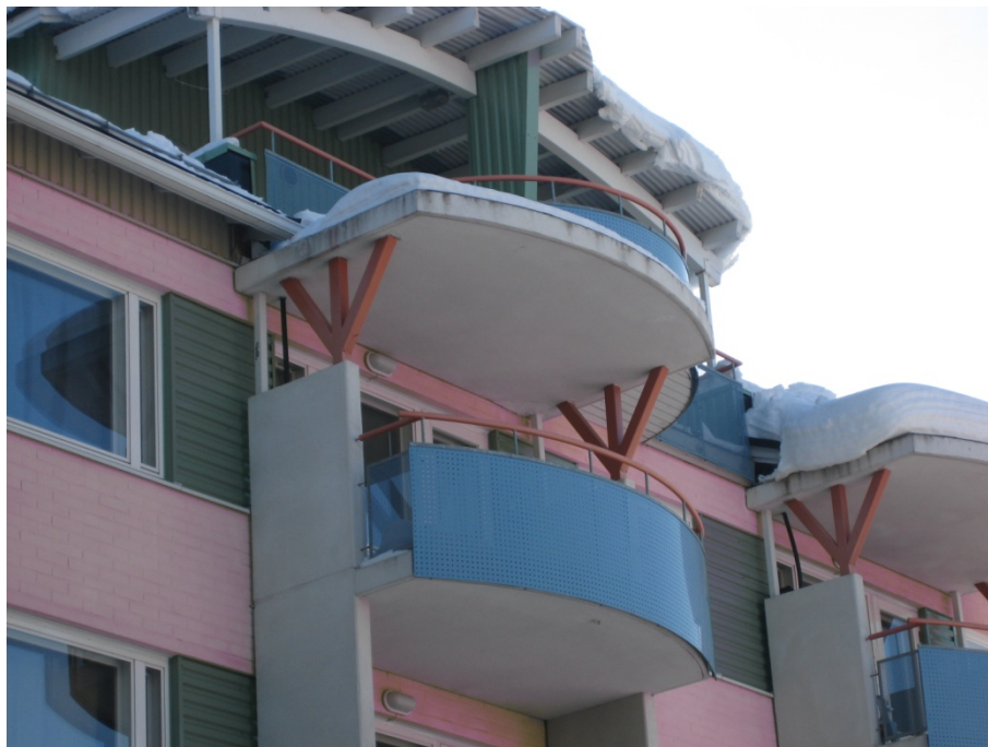
Figure 124. The neighbouring building DAS II after refurbishment. Photo: (Jyri Nieminen).
