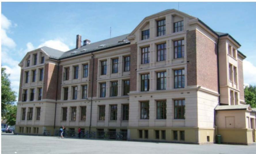
Figure 92. The main building of Strømsø School. Photo: (Drammen Eiendom KF).
