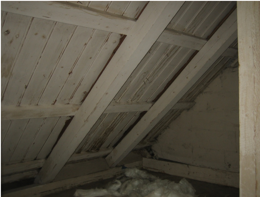
Figure 101. The roof seen from the cold attic. Photo: (Anders-Johan Almås).
