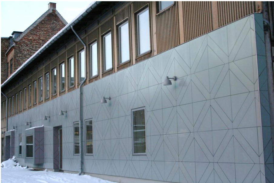
Figure 71. Partly insulation of the back of the Osram building. Photo: (Kim Haugbølle).
