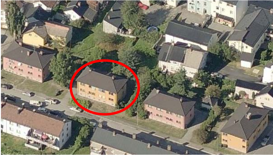
Figure 94. Aerial photo of case buildings. Photo: (Drammen Eiendom KF).
