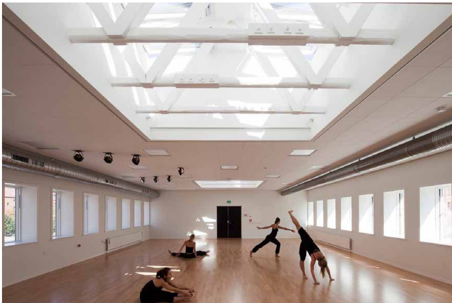
Figure 69. First floor of the renovated Osram house. Note the thick walls and comparably small heaters (for the room size). Photo: (Velux A/S).
