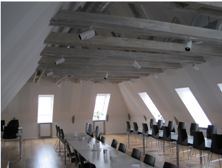
Figure 81. The canteen was moved from the cellar to the top floor as part of the renovation of the building. Photo: Ib Steen Olsen.
