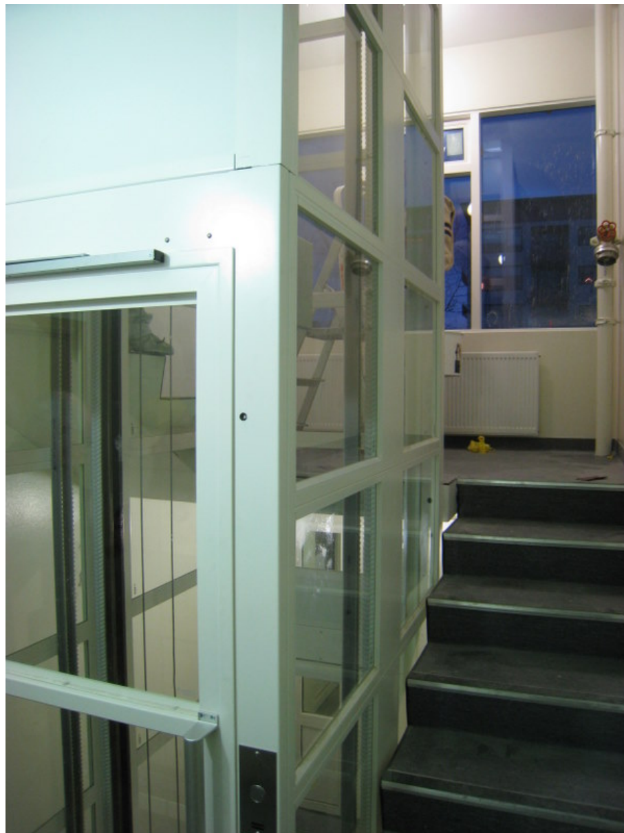
Figure 110. Existing staircase with an elevator built in. Photo: (Björn Marteinsson).
