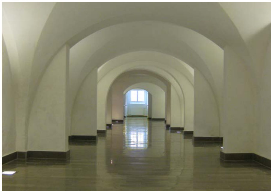
Figure 82. The refurbished hallway in the basement. Photo: Provided by Torben Kristiansen.
