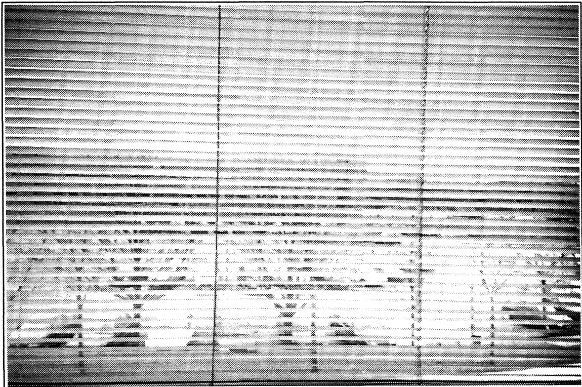
Figure 6.51 Interior photograph of the Venetian blinds with downward tilted slat angle ( VB +30^\circ ), showing the view-out function at a distance approximately 2 m from the window.
