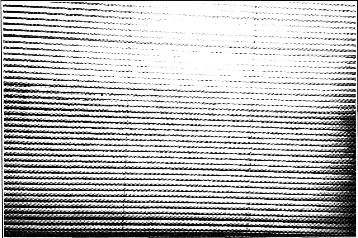
Figure 6.50 Interior photograph of the Venetian blinds with upward tilted slat angle ( VB -30^\circ ), showing the view-out function at a distance approximately 2 m from the window.
