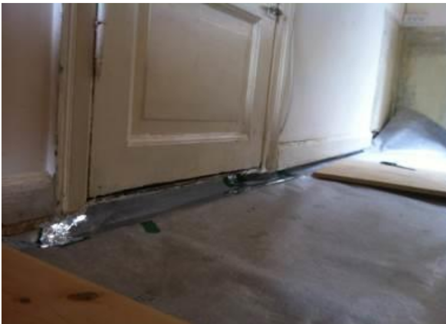
Figure 18 installation of the sealing membrane (cTrap)
