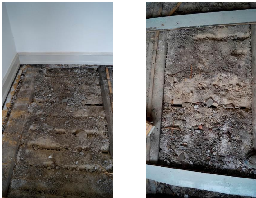
Figure 17 condition of wooden flooring during the renovation
