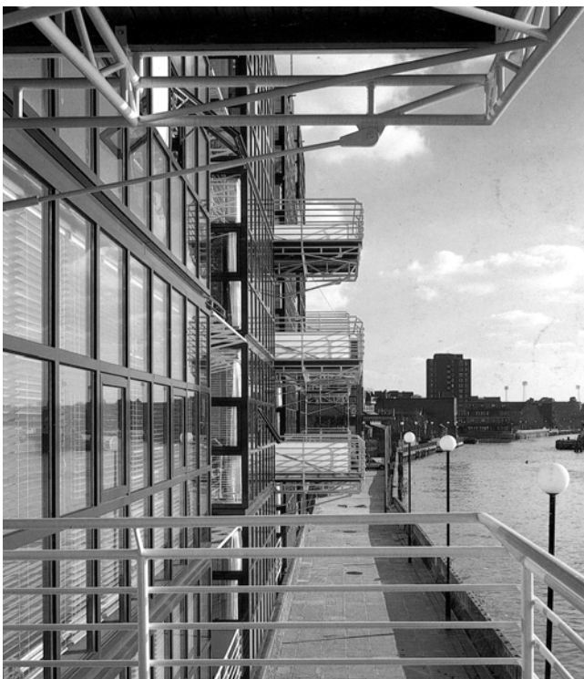
Boligbebyggelse: Thames Reach Housing, 1984-1987 Thames Wharf, Hammersmith, London Arkitekt: Richard Rogers.
