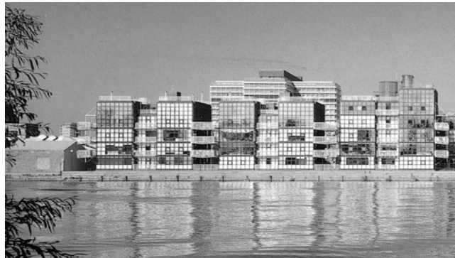
Boligbebyggelse: Thames Reach Housing, 1984-1987 Thames Wharf, Ham- mersmith, London Arkitekt: Richard Rogers.
