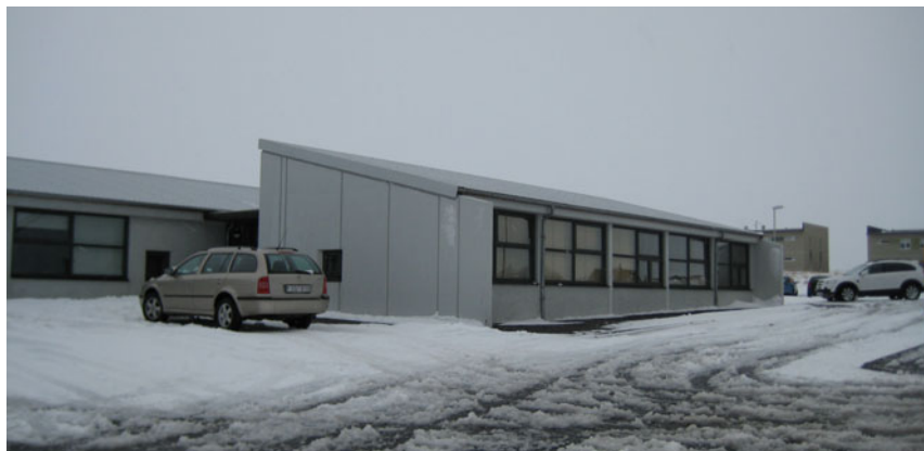
Figure 22. Holt nursery school building.
