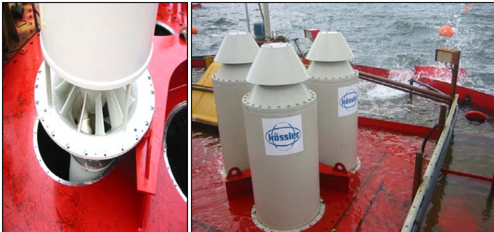
Fig. 4.13 Installation of draft tube and installed turbines.
