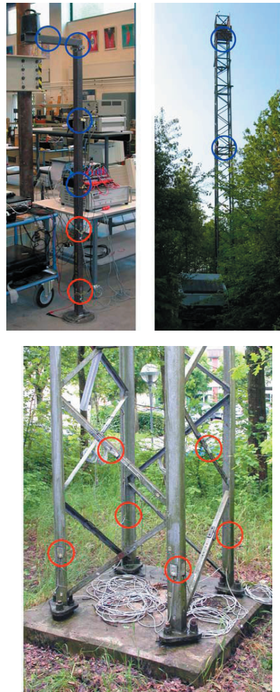
Figure 1. (Top left) Laboratory structure, (top right) lattice pylon, (bottom) base of lattice pylon. Red and blue circles indicate location of strain gauges and accelerometers respectively.
