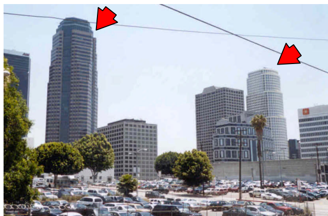
Fig. 1 Panoramic view of the buildings studied (Left: 52-storey; Right: 54-storey)
