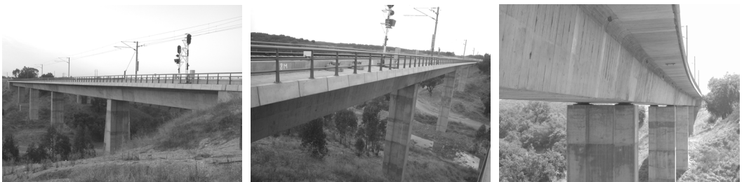
Figure 3 General views of Corona bridge
