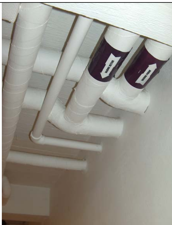
Insulated heating distribution system in basement.
