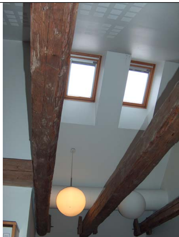
Windows with integrated solar shading.
