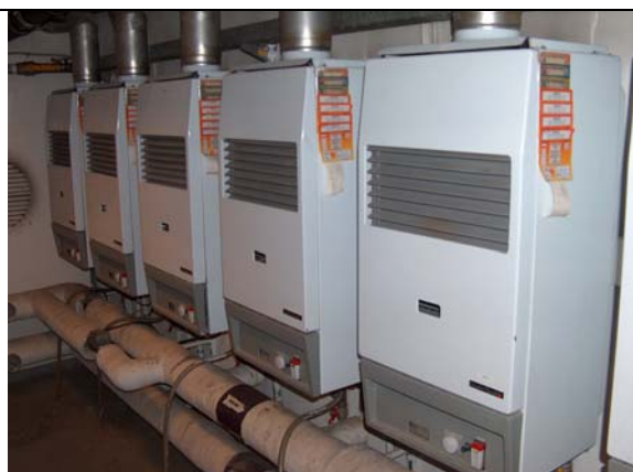
Natural gas boilers operating in cascade.
