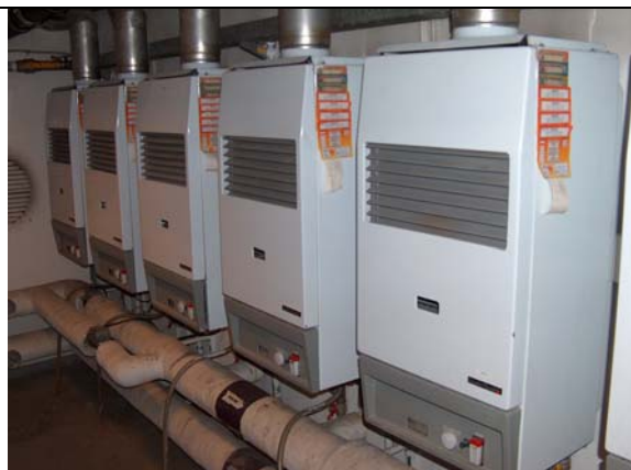
Natural gas boilers operating in cascade.
