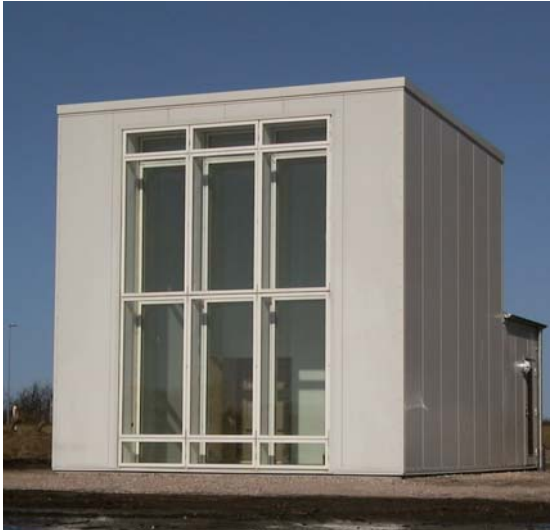
Figure 1. The “Cube”, outdoor test facility at Aalborg University.
