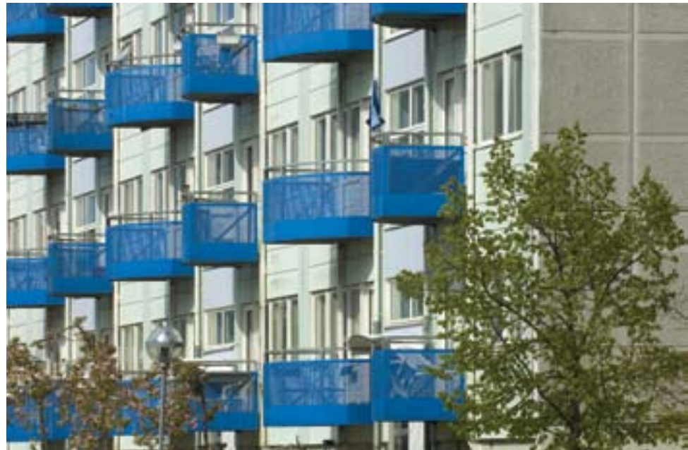
Renewal of worn-down housing areas
