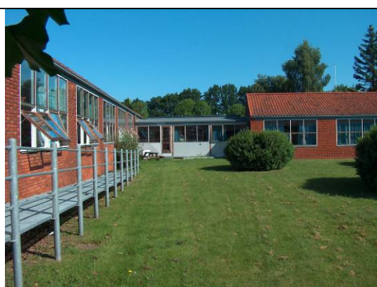
Connection building with media facilities.
