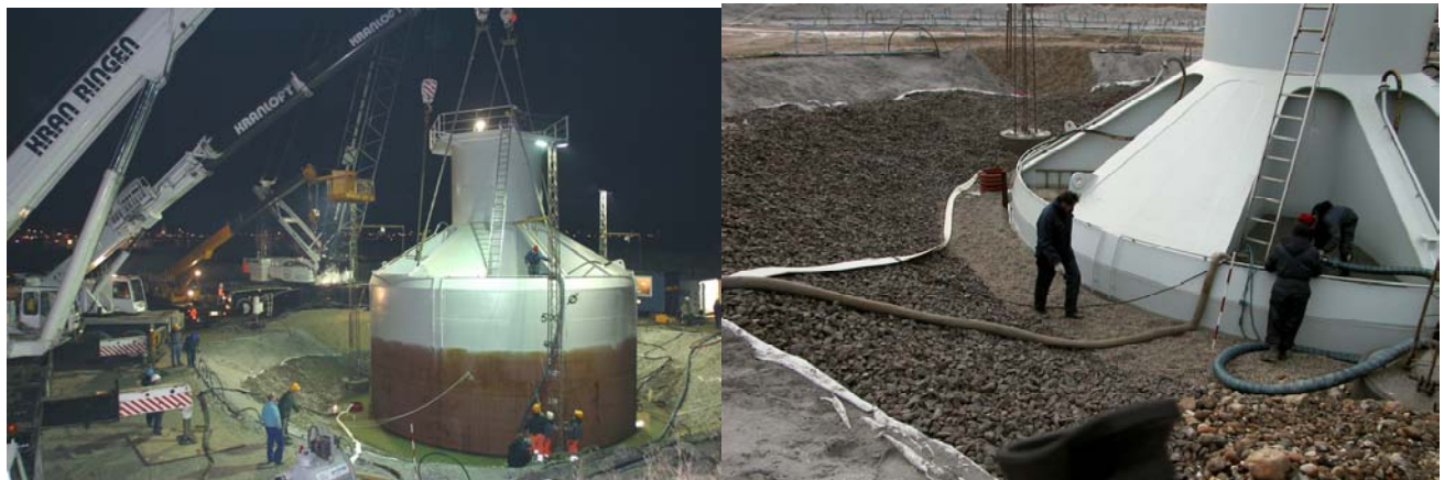
Figure 3: Installation of the prototype in Frederikshavn by suction. a) before installation. b) after installation .
