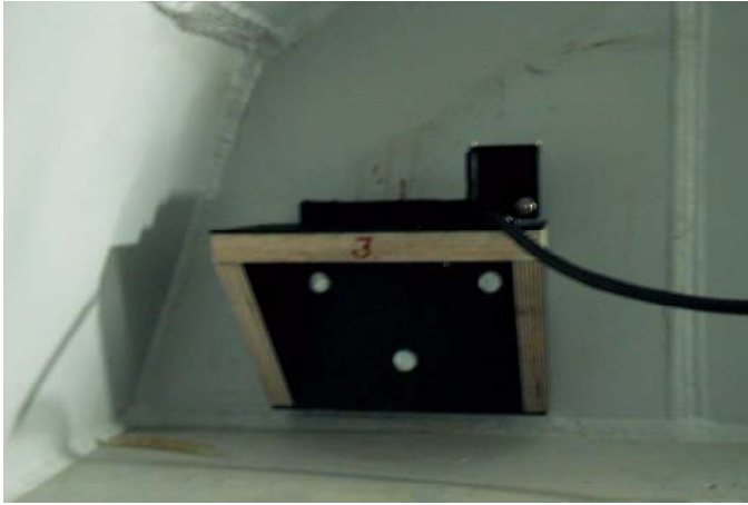
Figure 11. Accelerometer mount in the bucket near the skirt.
