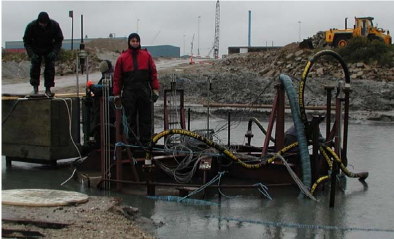
Figure 6. The 4x4 meter test bucket successfully installed.
