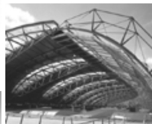
Geometrical relations construct associative geometrical modelling, represented through the system setup design by Grimshaw for the Waterloo station, United Kingdom, as a respond to a complex changing curvature.
