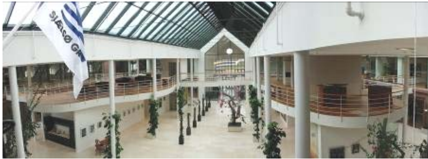
Ny Allerødgård naturally ventilated office building and atrium, HQ for Sjælsø Gruppen (major Danish developer company).
