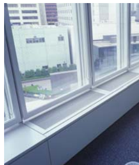
Figure 2.10b. Air Supply Swindow (View and detailed crossection)
