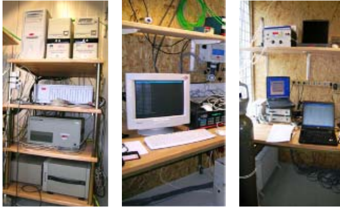
Figure 5. Equipment in the instrument room.
