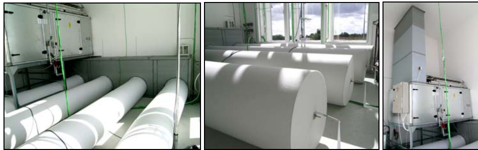
Figure 4. Ke-low impulse ducts (left, centre). Ventilation system in the experiment room (right).
